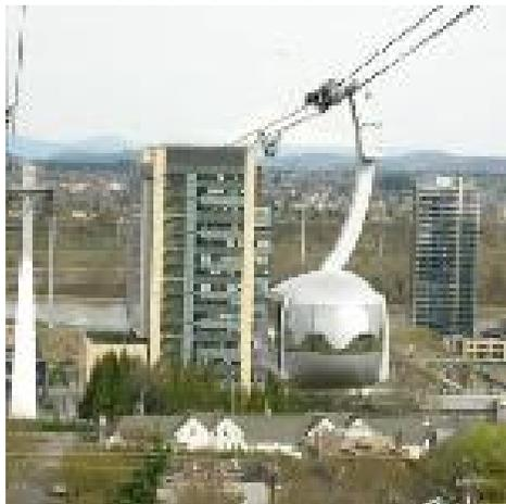
The Tram cabins travel 3,300 linear feet between the South Waterfront terminal adjacent to the Oregon Health & Science University (OHSU) Center for Health & Healing, and the upper terminal at the Kohler Pavilion on OHSU's main campus. Traveling at 22 miles per hour, the Tram cabins rise 500 feet for the three-minute trip over I-5, the Lair Hill neighborhood and the Southwest Terwilliger Parkway.
